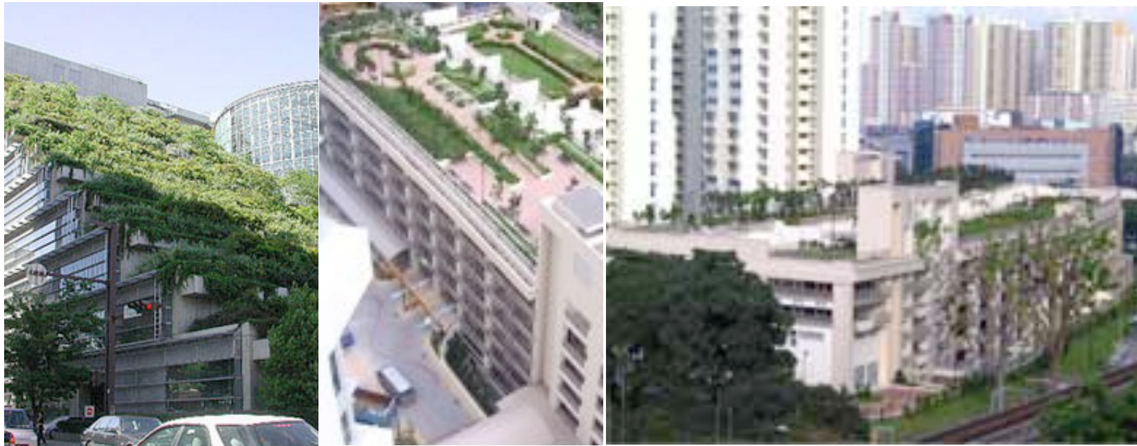
Parking Block Roof Garden, Queenstown, Singapore
